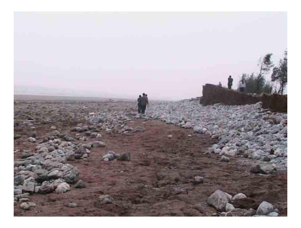
Erosion has started on another old sea dike, despite the rock armour and this old dike was washed away during last year typhoon season
