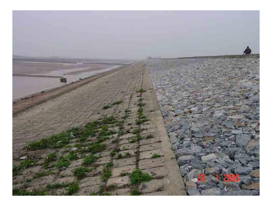
But this new dike, heavily protected by the extremely expensive rock armour, its inside batter was not protected, cover only by local vegetation, mostly weeds
